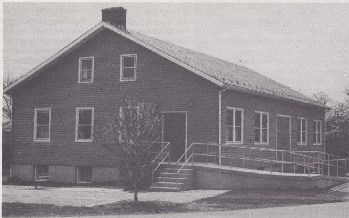
Holly House — GCNJ Headquarters
